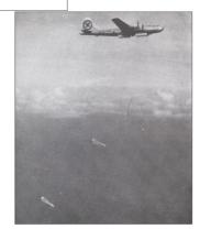
laying procedure is the same as bombing procedure number of mines carried is equal to saturation bombing rating or twice level b aircraft must be at very low altitude - no Norden bombsight
